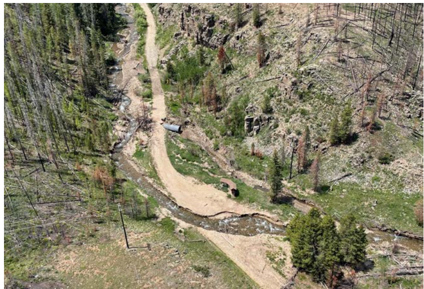
Road Blowout in Cabin Creek in the East Troublesome Fire Area 2022
